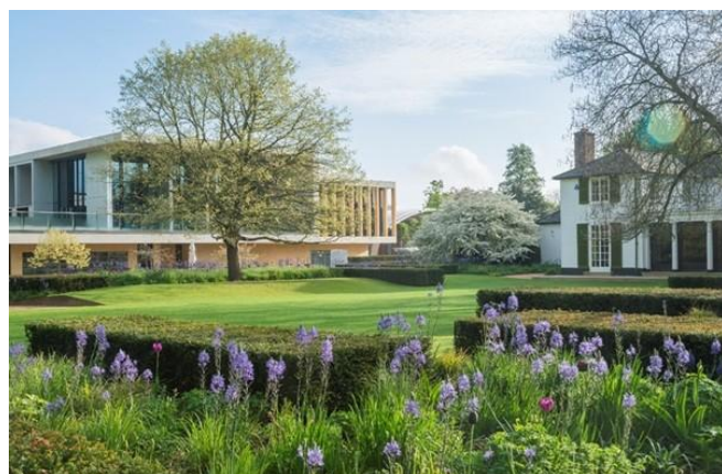
The Sainsbury Laboratory, which is located within CUBG and houses the Library and Herbarium. Talks and panel discussions will take place in the Sainsbury Laboratory Auditorium, and workshops will take place in the lab's breakout spaces. Image credit: Howard Rice.
